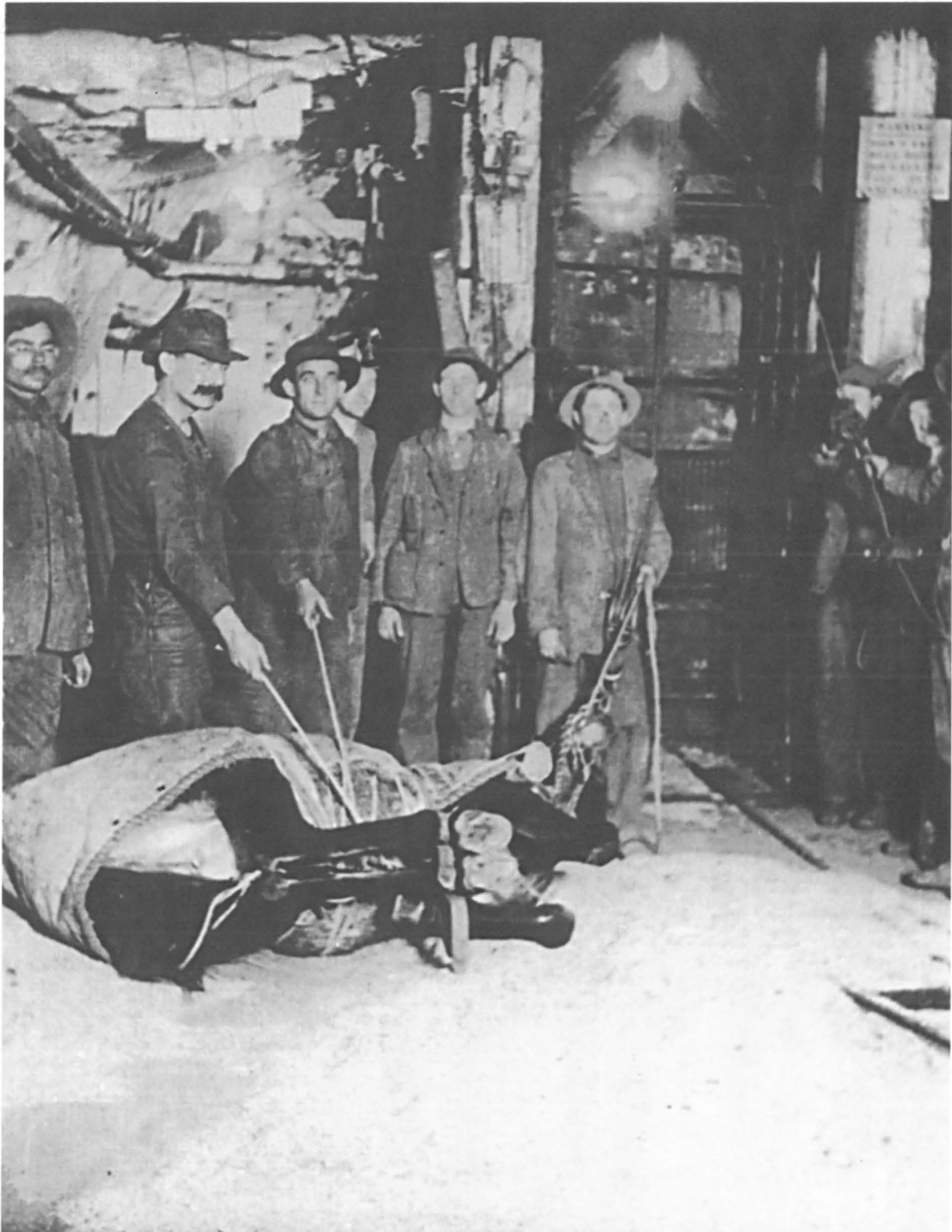
Getting mules into the mine was a major undertaking. To keep the animals from hurting themselves during transport in the small shaft and cage compartments they were securely wrapped in this canvas sweater, bound and hoisted into the cage shown in the background. Once underground, where this picture was taken, the wraps were removed and the mule released into his new environment. As indicated by the attendees present, moving the mules was a labor intensive effort. Note that in this photo one of the miners is wearing a carbide lamp. However, the shaft and station area are being illuminated by electric lights. Courtesy H. Mason Coggin Collection.
