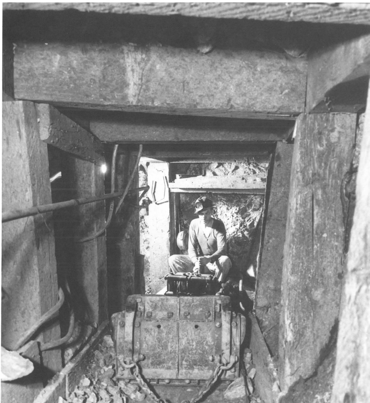
Slushing ore underground, Magma Mine, Superior. Courtesy of Magma Copper Co.
