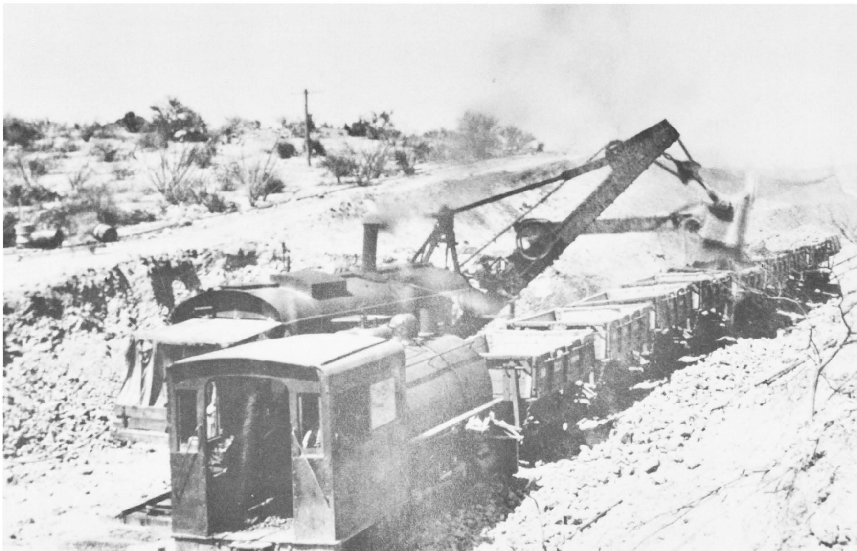
Constructing the road bed for the Gila Valley & Northern Railway, between Bowie and Globe. Courtesy of the Arizona Historical Society/Tucson.
