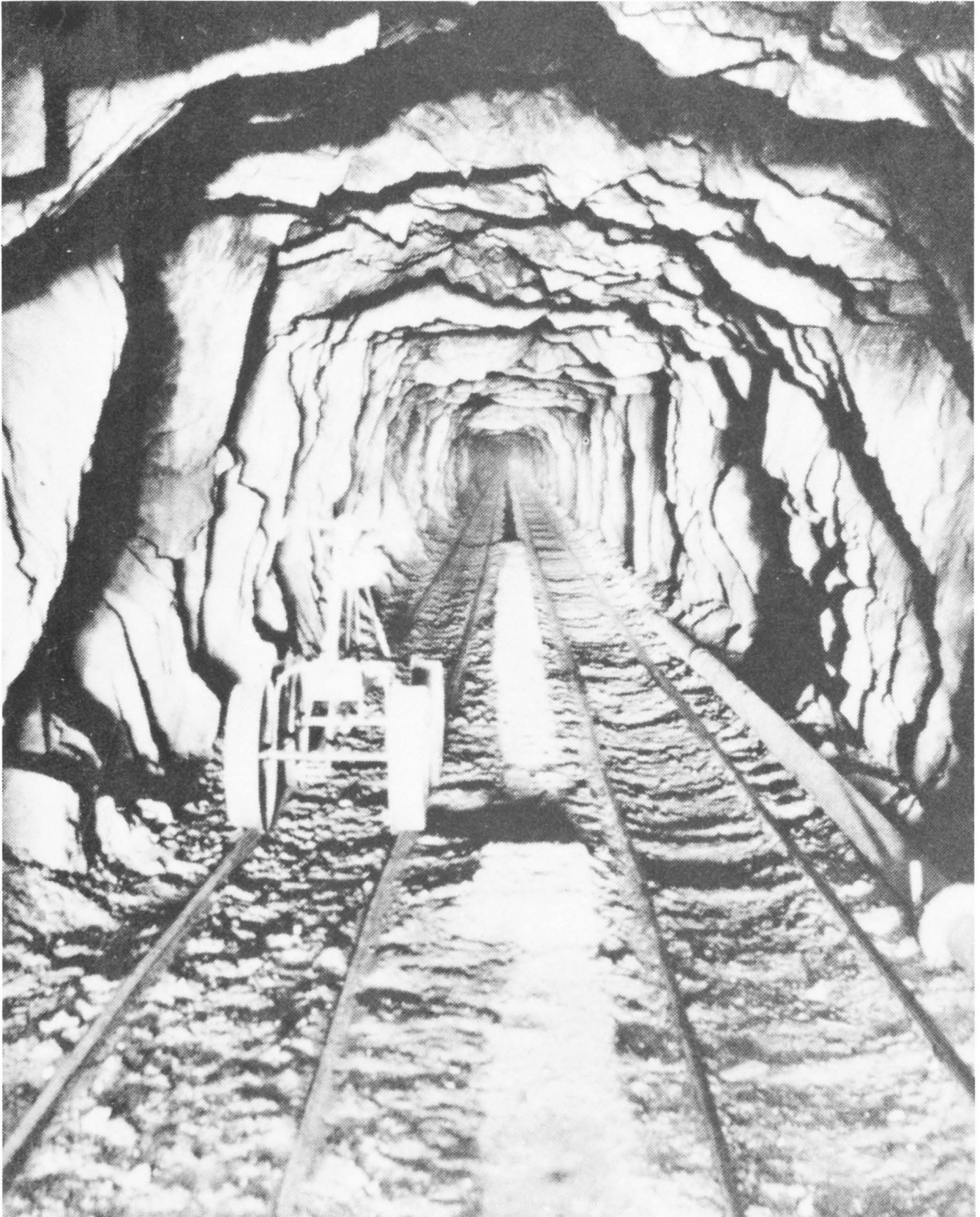
Double, narrow-gauge track of the Sheldon Mining Co. in the Poland Tunnel. Completed in 1904, the tunnel is 8,017 feet long. Courtesy of the Arizona Historical Society/Tucson.
