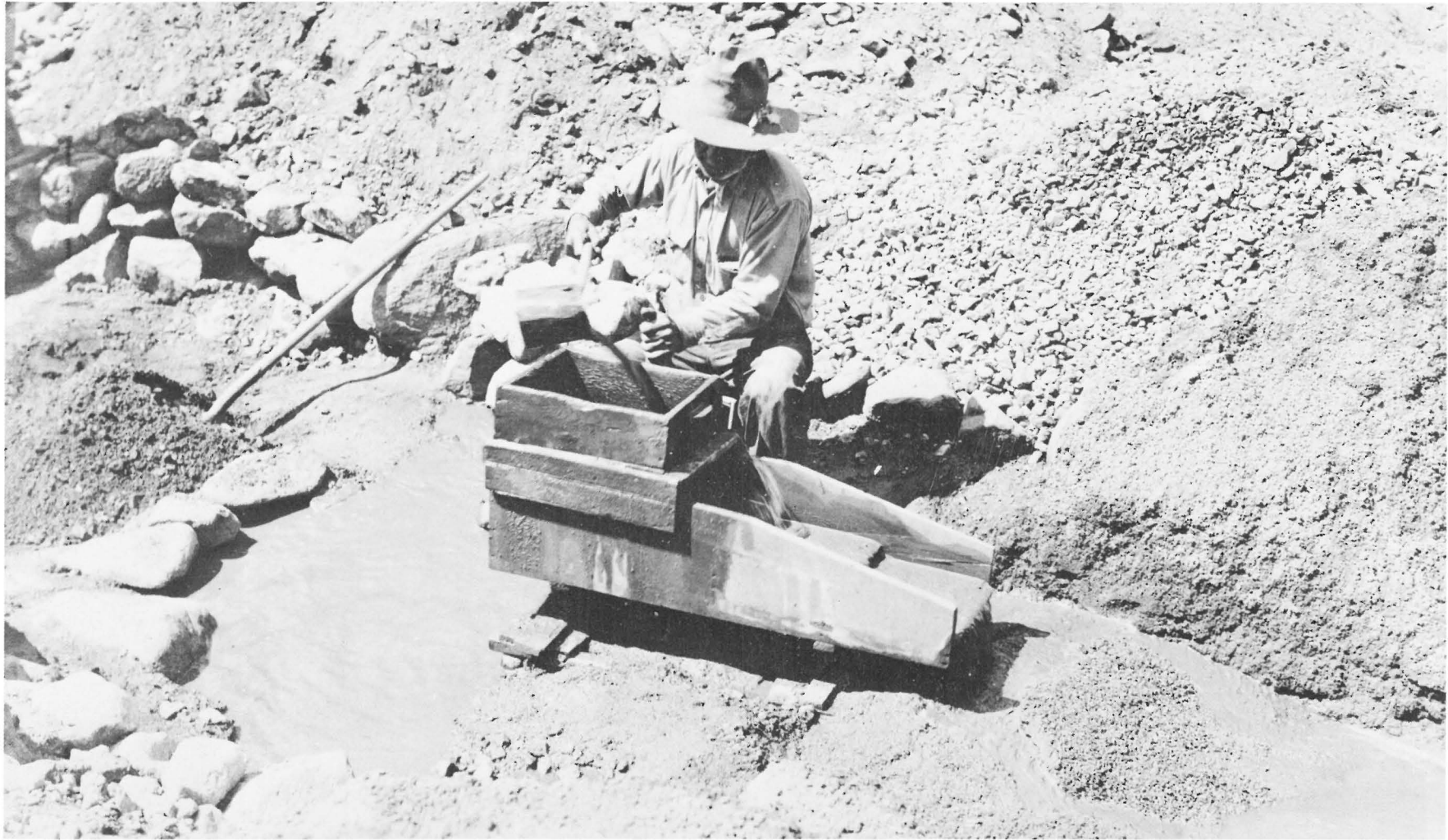
Placer miner operating a rocker in Copper Basin Wash. Fifty to sixty individuals operated rockers and small sluices in the drainage during the Depression. Courtesy of the Arizona Geological Survey.
