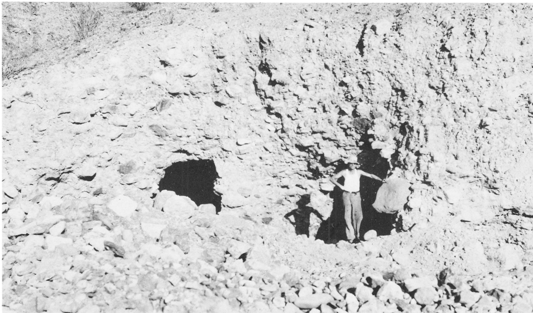
Tunneling on bedrock at the Sandy Harris placer, above the Colorado River at Willow beach, c. 1933. Ancient stream bar contains poorly sorted aggregate. Courtesy of the Arizona Geological Survey.
