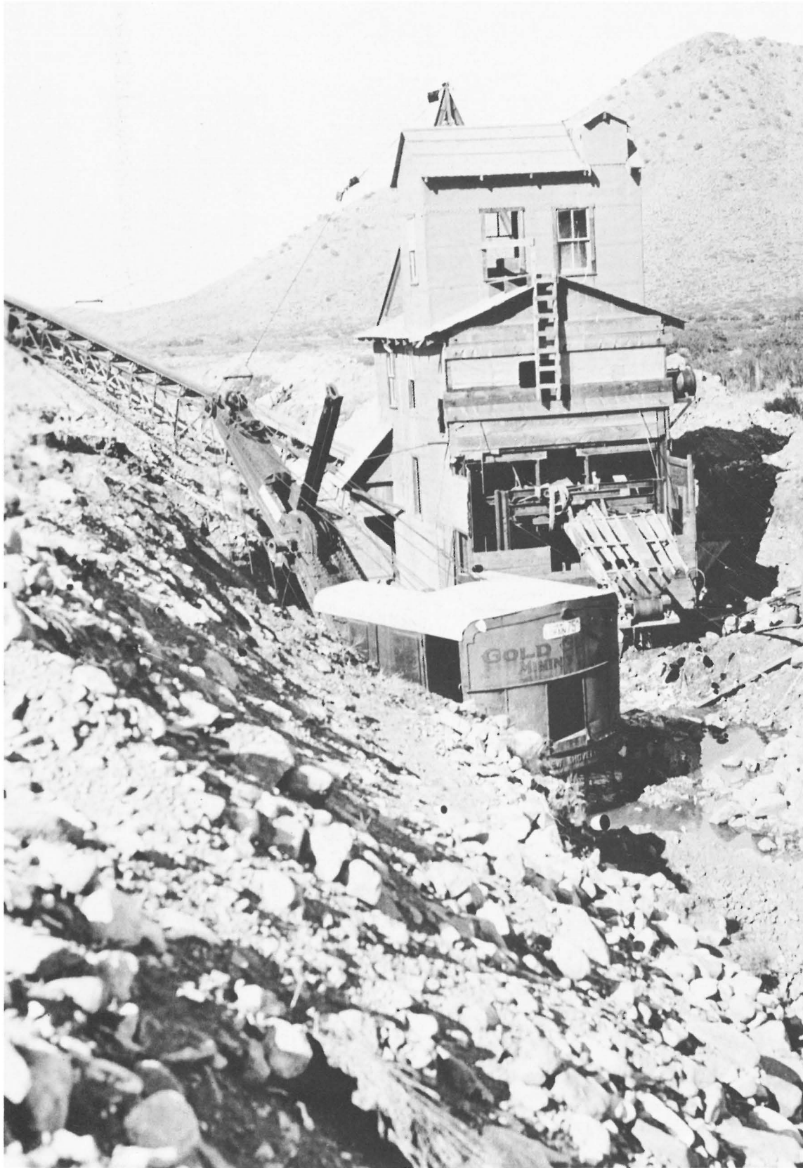
Dry-land dredge of the Gold Gulch Mining Co., Teviston district, 1933. Rated capacity was 50 cubic yards per hour. Courtesy of the Arizona Geological Survey.
