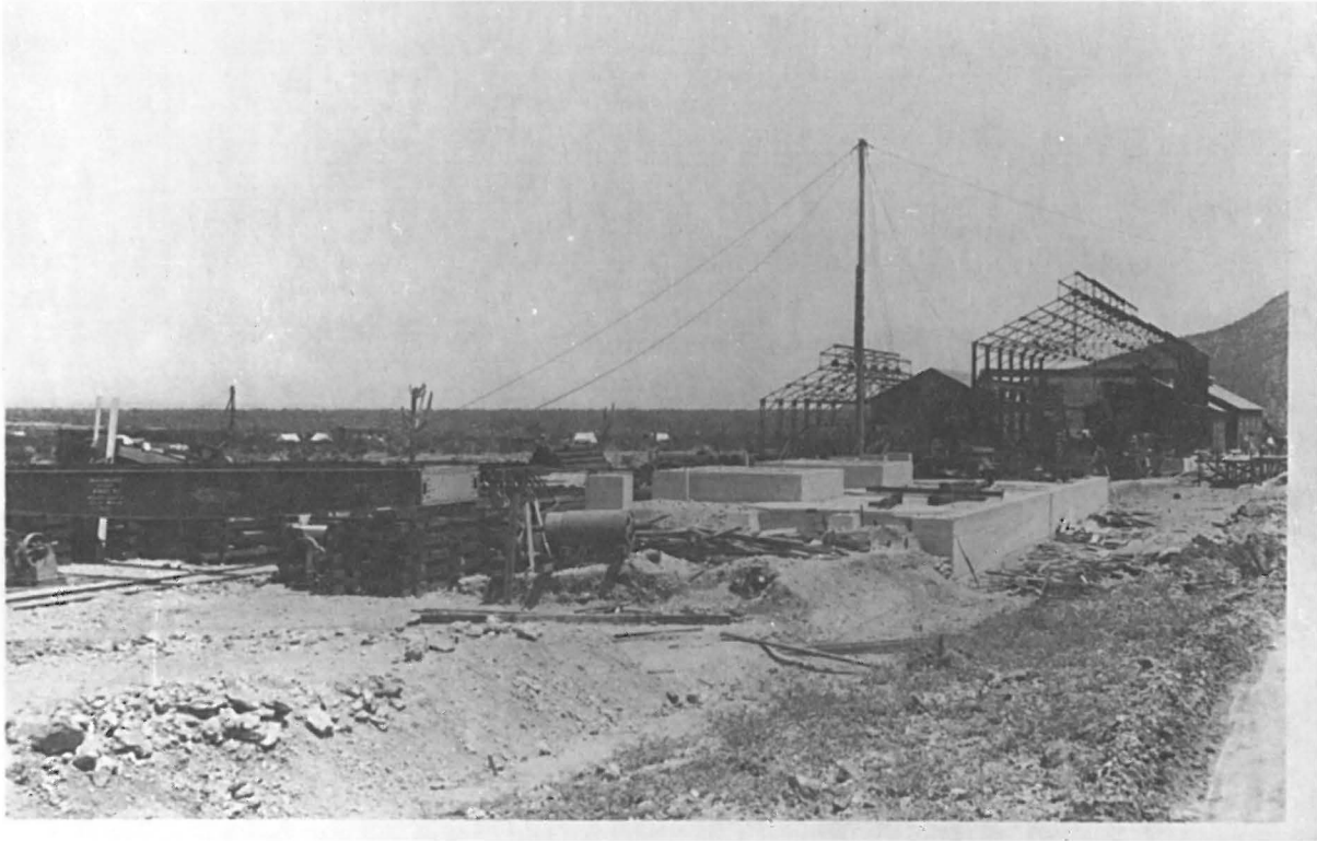
The foundations of the smelter during construction. The completed frame of the power plant and boiler house can be seen in the background. Photo courtesy of the University of Arizona, Special Collections.
