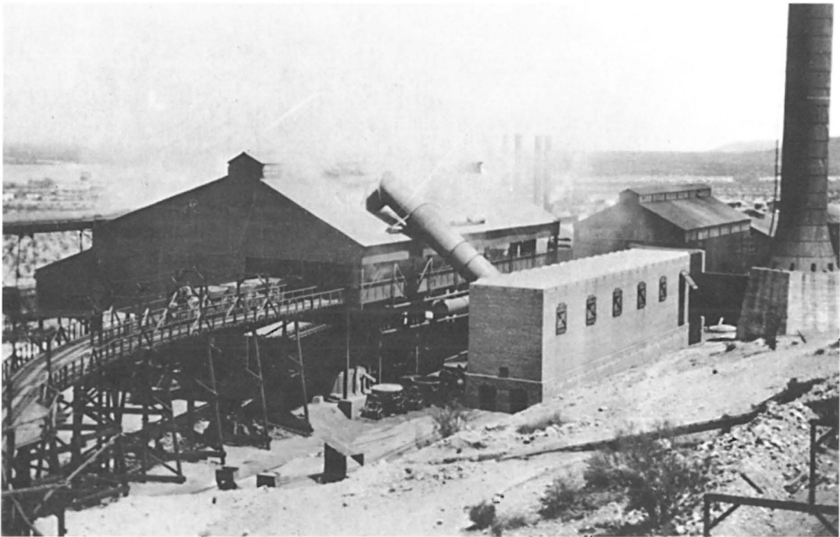
Close up of the smelter and dust chamber as seen from the ore bins. Note the slag pot being filled at the settler. Photo courtesy of the University of Arizona, Special Collections c1908.
