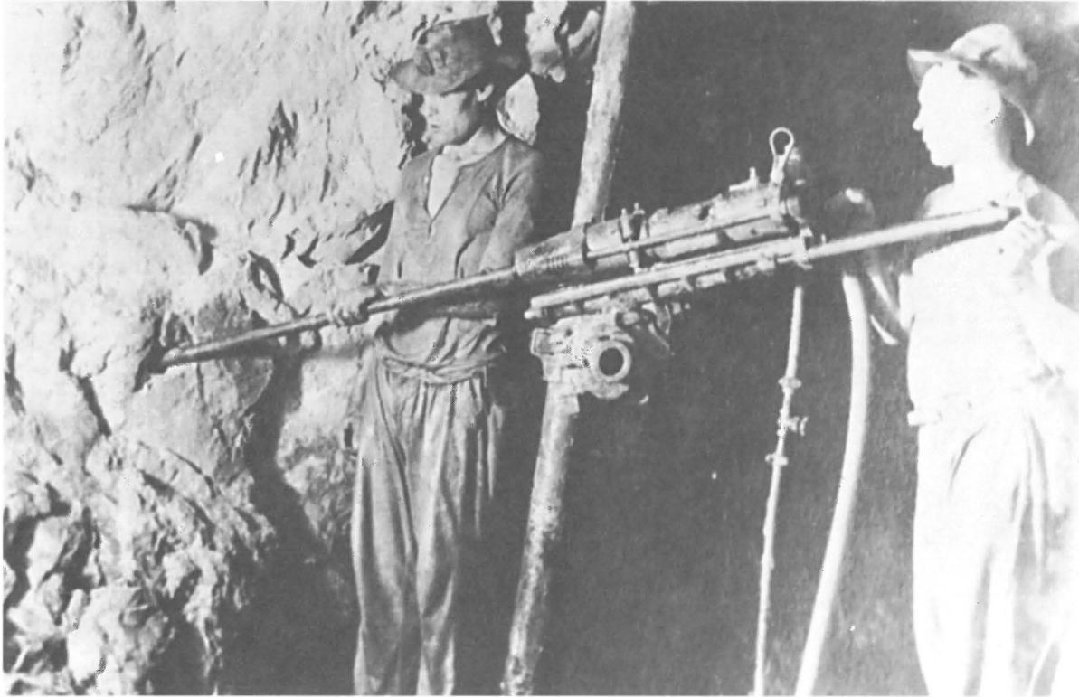
Waugh drilling apparatus, 1917. Courtesy of Gila County Historical Society.
