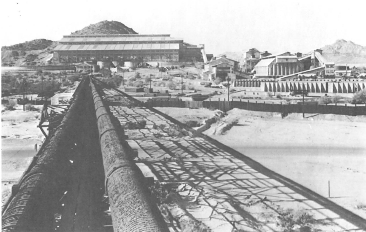
Photo taken November 27, 1939. In left background is the concentrator. To its right are the crushing plants and ore bins; in front of them are the leaching tanks. Wood-stave pipes coming from the concentrator are carrying sulfide ore tailings to the tailings disposal area. Courtesy of the Phelps Dodge Corporation.
