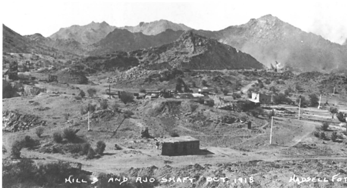
Compare with photo 2. Mining on Hill NO. 3 (October 1918). Ajo Shaft (center) was developed to check prospect drilling and to mine sulfide ore for the flotation process pilot plant; other shafts at left center were also for checking and to remove high-grade oxide ore mined in the glory hole. Courtesy of the Arizona Historical Society/Tucson, Hadsell Collection #64215.
