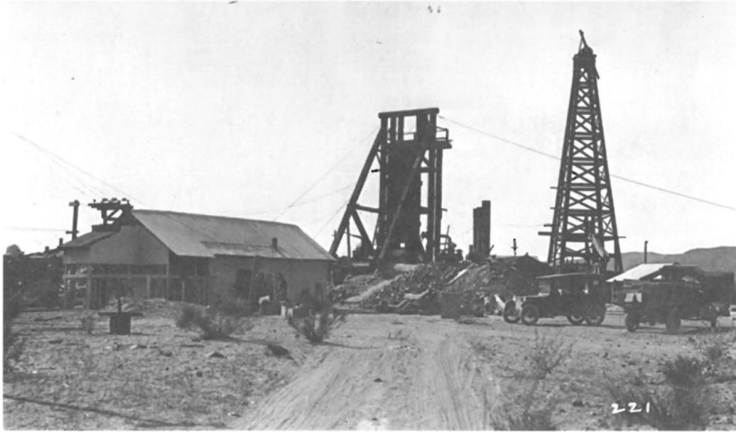
Well No. 1, six plus miles north of Ajo. Tower at right was the large oil-well drill rig that started to drill the water prospect hole in the Spring of 1913. To its left was the sinking headframe for the development shaft (100 feet south of the drill hole); started April 26, 1914. Courtesy of the Arizona Historical Society/Tucson, Buehman Collection #64221
