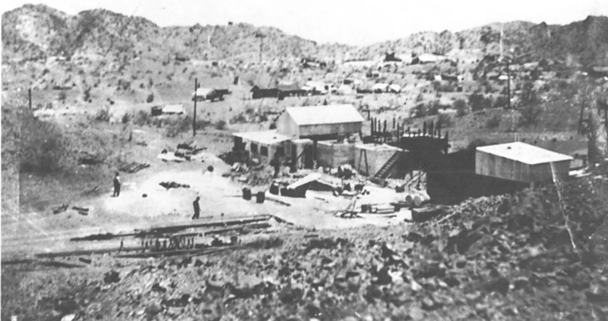
40-ton oxide-ore pilot plant under construction in "Old Ajo;" completed January 31, 1915. Courtesy of Ajo Historical Society/Tucson, Tobelmann Album #70267.
