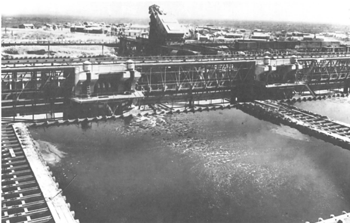
In the foreground is a leaching tank that has oxide ore and sulfuric acid leaching solution in it; beyond is the Hulett unloader which removed the leached tailings from the leaching tanks, beyond it is the town of Clarkston. Courtesy of the Arizona Historical Society/Tucson, Bevil Gordon Granville Collection #30485.
