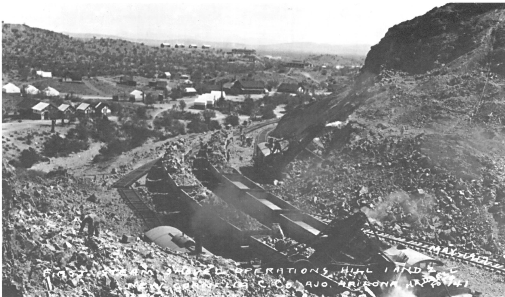
Steam shovels ining Hill No. 1 (on right) and Hill No. 2 (on left). There are two trains of ore cars. Left middle are single tent houses; above center are two larger tent houses. On the horizon are the four Department-Head Residences and the hospital (finished in 1919). Courtesy of the Arizona Historical Society/Tucson, Hadsell Collection #64141.
