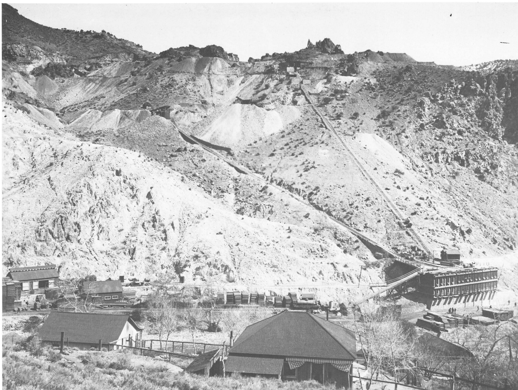
These are the Metcalf and Wilson Inclines connecting the Metcalf Mines with the storage bins and the Coronado railroad, c. 1917. Courtesy of Phelps Dodge Corporation.
