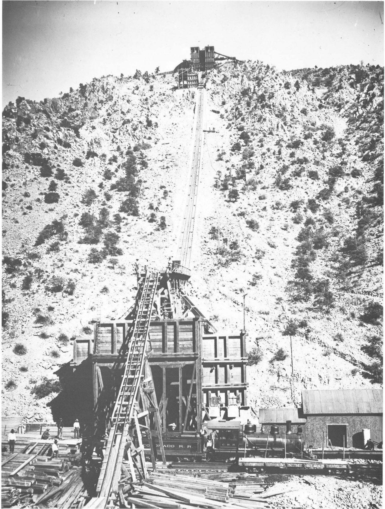
The Shannon Copper Company Mines were located near the top of this incline. Ore cars were lowered on the incline to the bins and Coronado railroad below. Later, the Shannon Company built their own railroad. Courtesy of Phelps Dodge Corporation.
