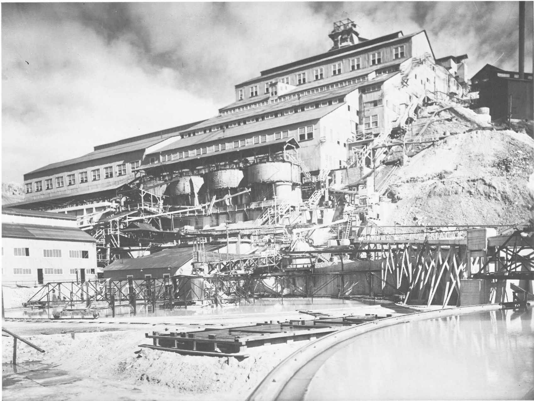
The Number 6 concentrator was built in Morenci by the Arizona Copper Company in 1906, to handle the lower grade sulfide copper ore from the underground Humboldt Mine. It remained in production until 1932, when all underground mining ceased. Courtesy of Phelps Dodge Corporation.
