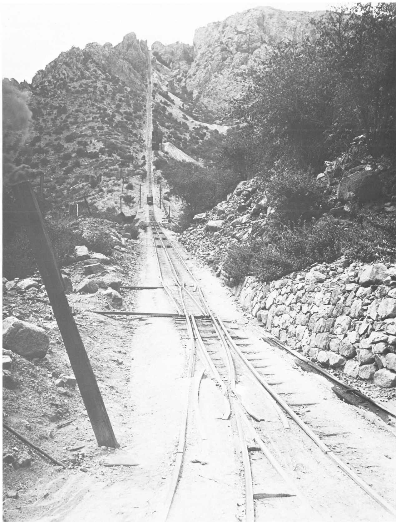
The Coronado Incline was the most spectacular in the district, connecting the Coronado Mine with the town of Metcalf, a difference of 1500 feet in elevation. Courtesy of Phelps Dodge Corporation.
