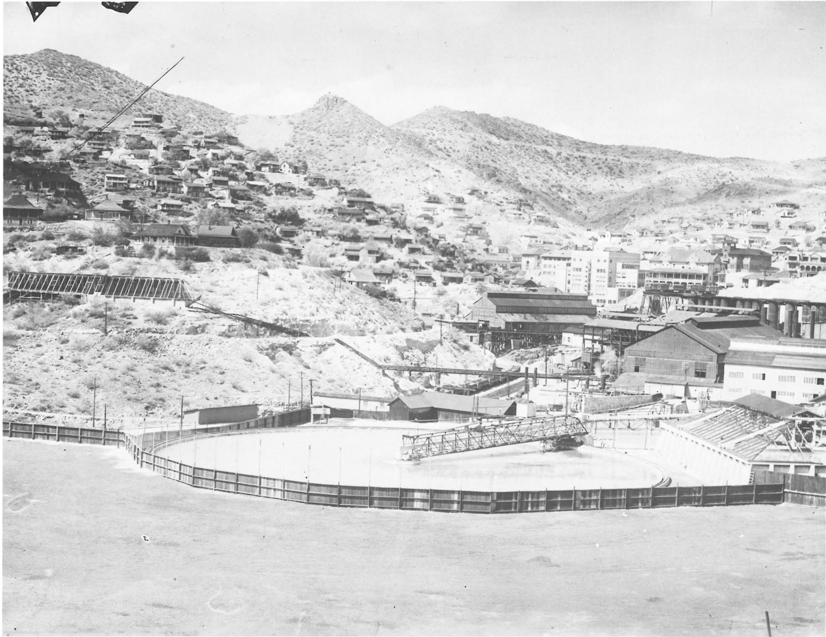
A thickener tank for the Number 6 concentrator appears in the foreground, and Morenci is shown as it appeared c. 1925. Courtesy of Phelps Dodge Corporation.
