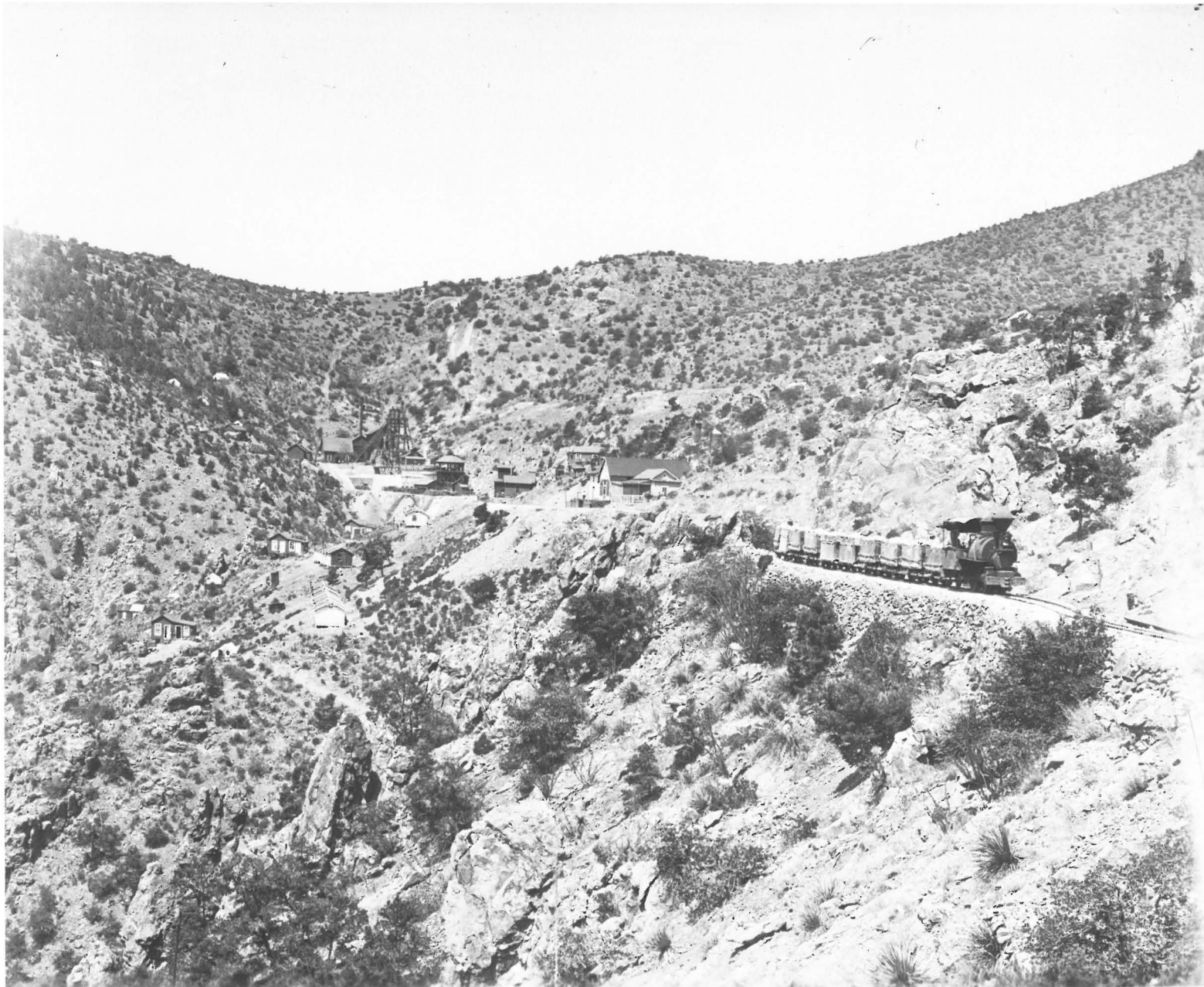
A small locomotive provides the power to move ore from the Coronado Mine to the top of the Coronado Incline. Courtesy of Phelps Dodge Corporation.
