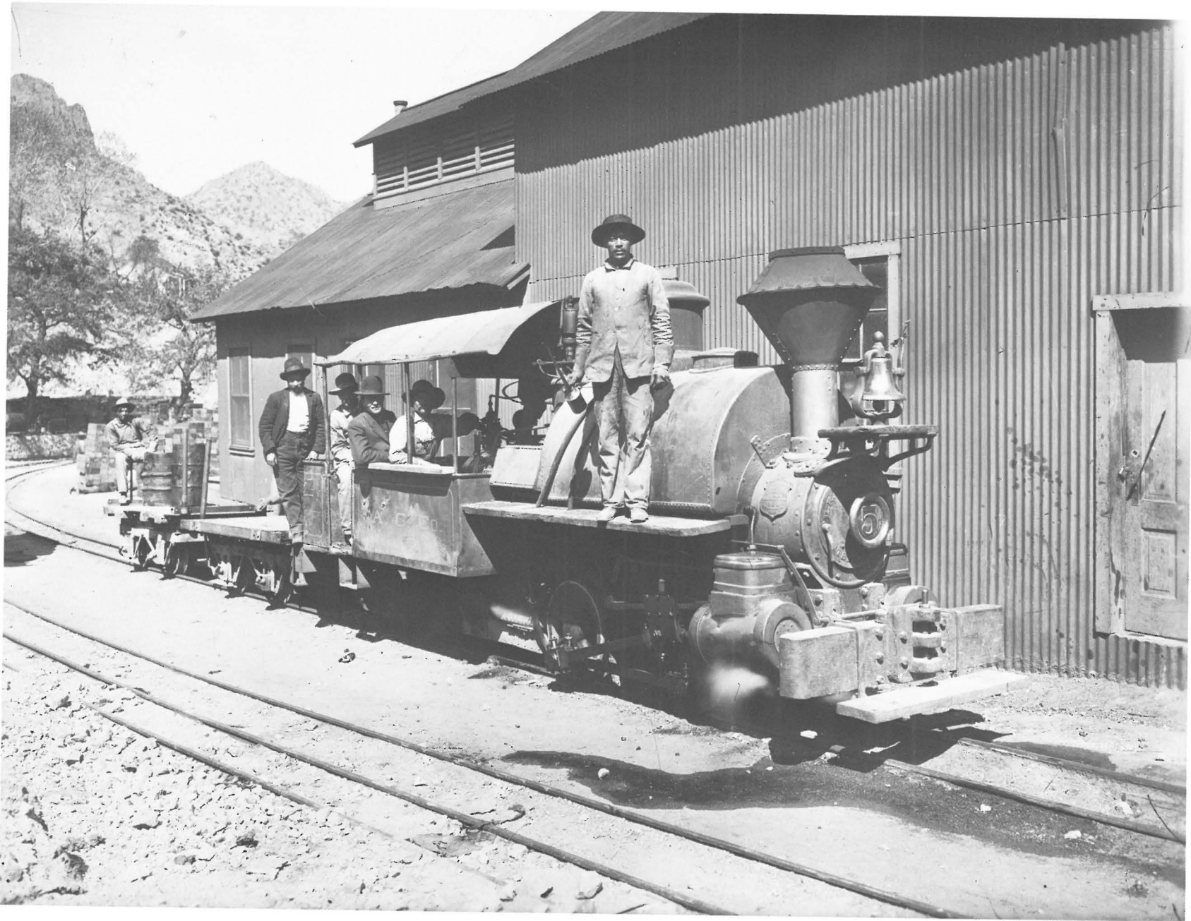
A baby gauge (20" between rails) locomotive on the Coronado railroad, by the engine house at Metcalf in the 1890's. Courtesy of Phelps Dodge Corporation.
